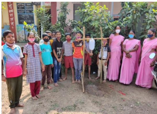
Hand washing station built by students and ASHA
